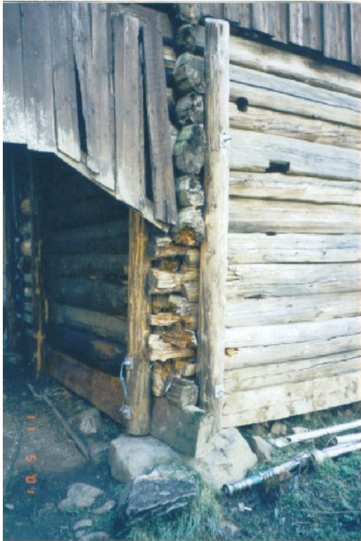
Photo 2.12: Double plank carriage seen from the outside on the barn at Bakken, Bjørgum.
