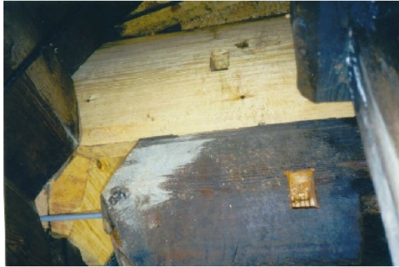
Photo 2.3: Using gjengestag to repair the cantilever (also called skakestokk and overmann and undermann ) on a loft at Dale, Valle.
