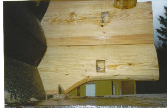
Photo 2.4: Installed cantilever on a loft at Dale, Valle.
