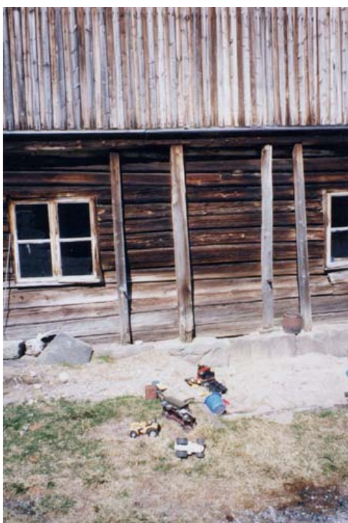
Photo 2.13: Plank carriage on an animal shed, Systog, Løyland, Valle.
