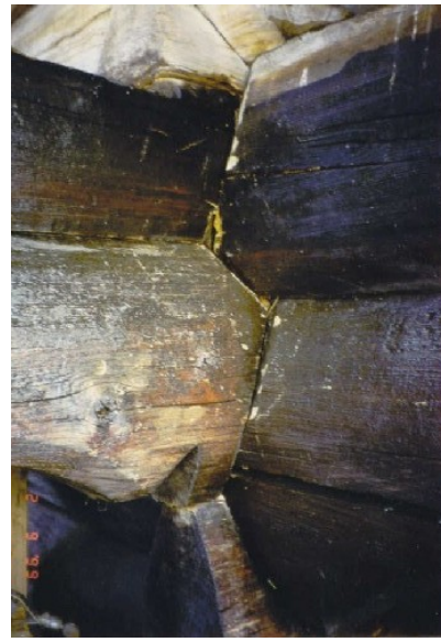
Photo 2.8: Finished repair at Bakken, Bjørgum, Hylestad.
