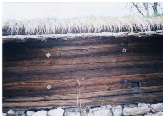
Photo 2.14: Plank carriage at Henriksentunet, Bykle.
