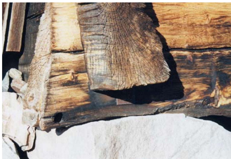
Photo 3.1: Securing a pushed-out sill at Rygnestadtunet, Valle.
