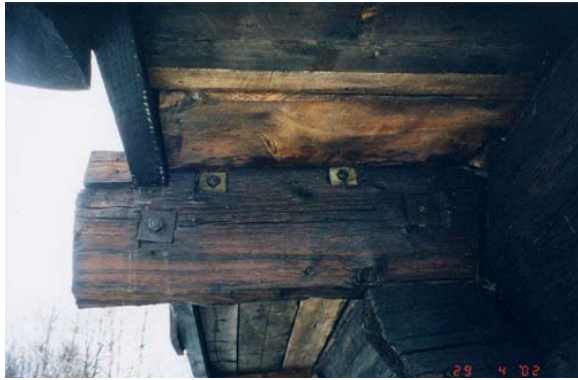
Photo 2.24: Strengthening of a rot-damaged cantilever on the balcony at Holslopte, Bykle.
