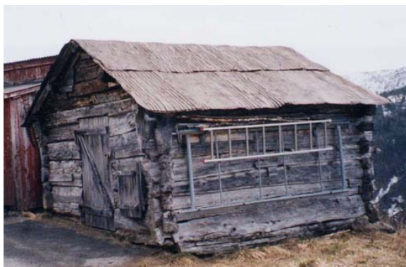
Photo 2.37: Pitch panels on a hut at Jåro, Bykle.
