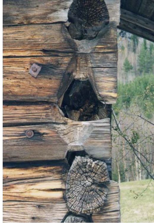
Photo 2.11: External plank carriage seen from the outside on the loft at Flateland.
