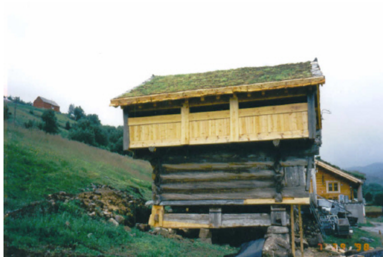
Photo 3.2. The loft Muggslopte, Bykle.
