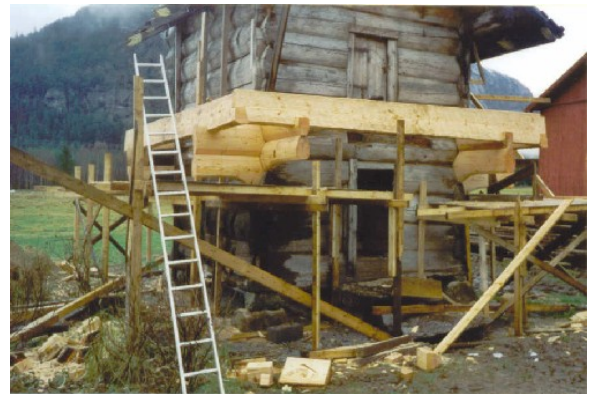
Photo 2.5: Everything installed with balcony sills (called svalesydd or tilemor ) in place on a loft at Dale, Valle.
