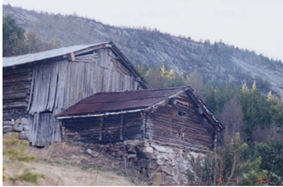
Photo 2.39: Pitch panels on an animal shed at Berg, Hylestad.
