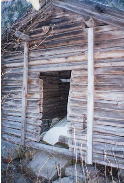
Photo 2.10: Interior and exterior plank carriage seen from the outside on the hut at Flåstrondi.
