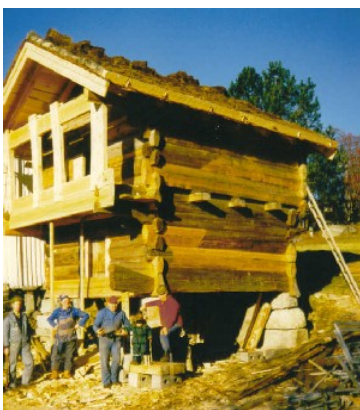
Photo 2.19: The loft Brottveitslopte restored according to antiquarian methods, Valle.
