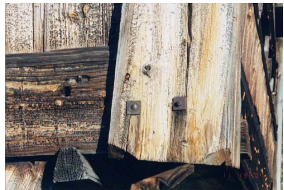
Photo 2.27: Securing a corner post on the balcony at Rygnestadtunet, Valle.
