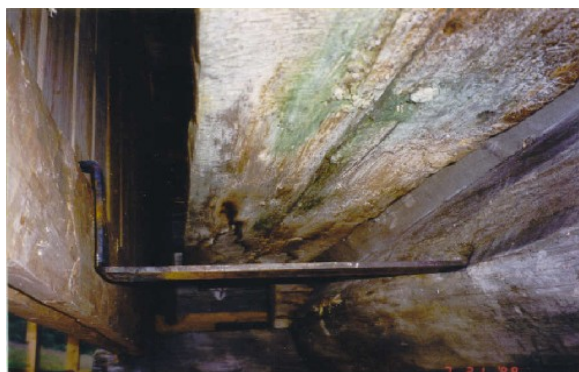
Photo 2.21: Iron binding used on Muggslopte, at Innestog, Byklum, Bykle.
