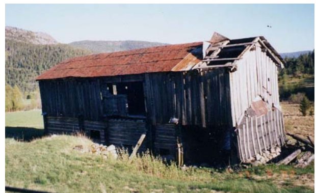
Photo 2.38: Pitch panels on a barn at Uppstad, Hylestad.
