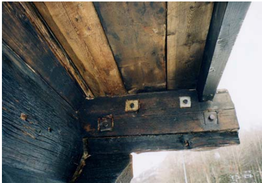
Photo 2.25: Strengthening of a rot-damaged cantilever on the balcony at Holslopte, Bykle.
