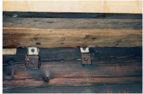
Photo 2.26: Strengthening of a rot-damaged cantilever on the balcony at Holslopte, Bykle.
