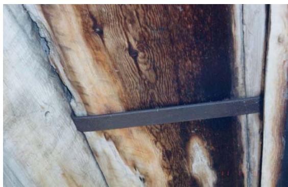
Photo 2.20: Securing floorboards on the balcony at Rygnestadtunet, Valle.
