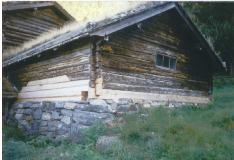
Photo 2.16: Antiquarian methods were used to restore the animal shed at Rygnestadtunet.
