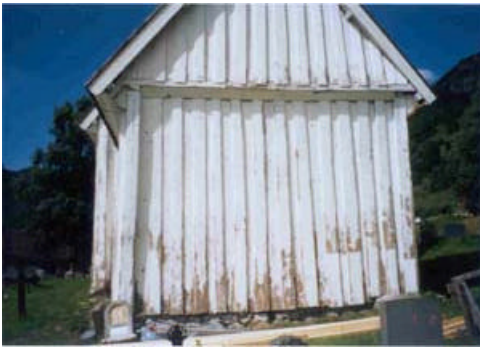
29. Chancel: Wall VIII. Hand-forged nails used to tighten lose panels. Scraped and painted.
