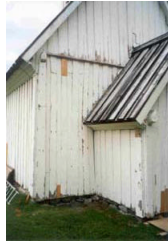
23. Nave Gable - end walls: Wall CCC. External panels were replaced. Photo shows the use of new materials. Scraped and painted.
