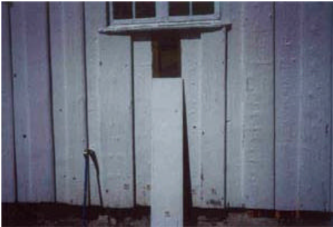
27 og 28. Chancel: Wall VI. Dismantled the foundation wall to examine the joists and floorboards. The joists were lying in dry boggy soil with minor rot damage. The joist foundations were straightened up. The foundation wall was replaced on crushed rock. Scraped and painted.
