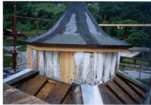
43. Roof: There was large rot damage on the roof panels. There were no damage to the nailing strip. The ridge of the roof was covered with sink (replaced existing sink). The same pattern for drainage was used as before.
