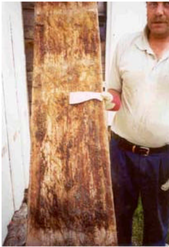
35 og 36. Chancel: Wall YC. Some panels were turned around. There were visible evidence of tar treatment and use of wooden nails.
