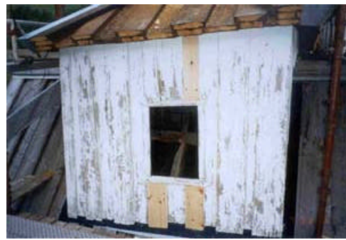
41. Bell tower: The church bell tower was scraped and painted. Photo shows use of new materials.
