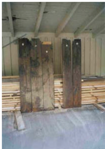
5. Entrance vestibule: Photo number 5 shows the new floor boards, the old ones had been replaced earlier.
