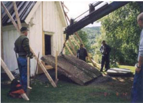
9. Stairs: The flagstone in front of the door is the original, the flagstones lie in crushed rock.
