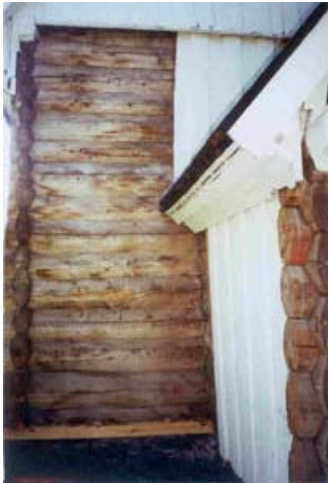
22. Nave Gable - end walls: Wall CCC. The sill was bunged up with new material and the wall was replaced.
