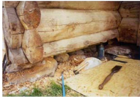
21. Nave Gable - end walls: Wall CCC. Dismantled the foundation wall and external panels. The sill was rot damaged.
