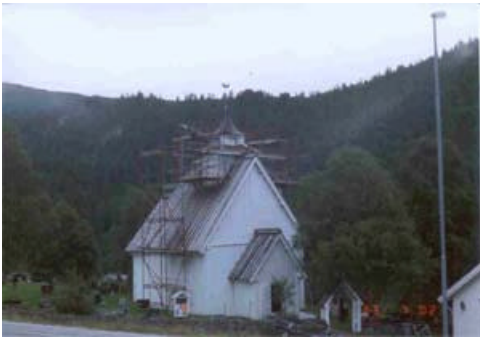
40. Bell tower: The detached scaffolding was built by Ivar Pedersen, Tveit.
