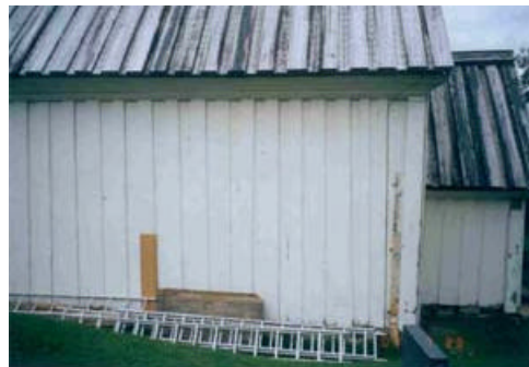
19. Nave Gable - end walls: Scraped and painted Wall CCCC.
