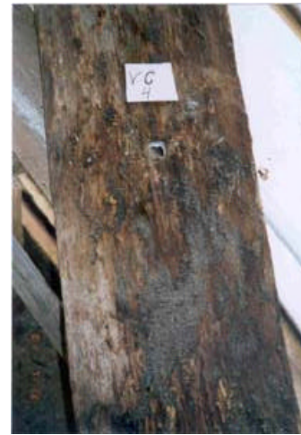
35 og 36. Chancel: Wall YC. Some panels were turned around. There were visible evidence of tar treatment and use of wooden nails.
