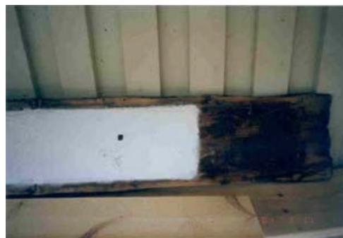
34. Chancel: Wall YC. Photo shows one panel fixed with wooden nails.
