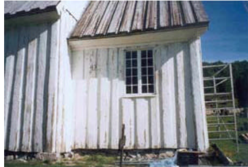
27 og 28. Chancel: Wall VI. Dismantled the foundation wall to examine the joists and floorboards. The joists were lying in dry boggy soil with minor rot damage. The joist foundations were straightened up. The foundation wall was replaced on crushed rock. Scraped and painted.
