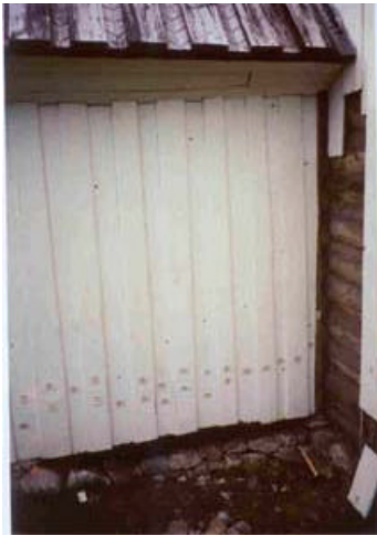
7. Entrance vestibule: Wall II was scraped and painted.
