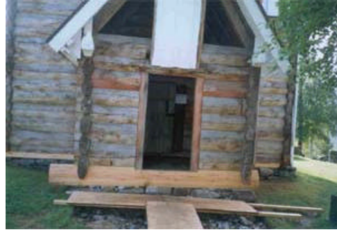
2. Entrance vestibule: Reconstructed the sill and joined it in place.
