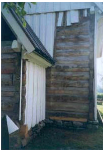
9. Stairs: The flagstone in front of the door is the original, the flagstones lie in crushed rock.
